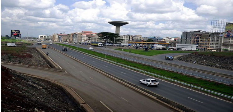
A completed section of the Outer Ring Road in Nairobi
