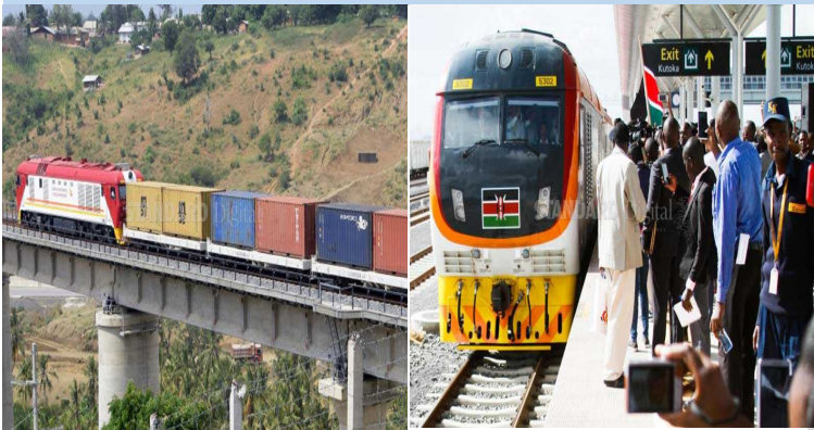
The SGR phase one completed and operational
