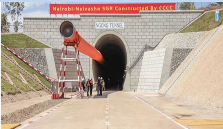
Ngong Tunnel of SGR Phase Two; SGR Phase 2 (Nairobi to Naivasha) has received an allocation Ksh.55.8bn
