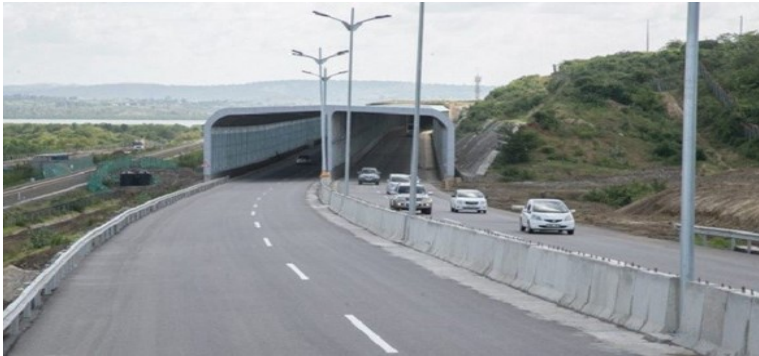
A completed section of Dongo Kundu bypass in Mombasa
