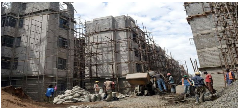
Construction of 2,720 affordable housing units at River Estate Ngara
