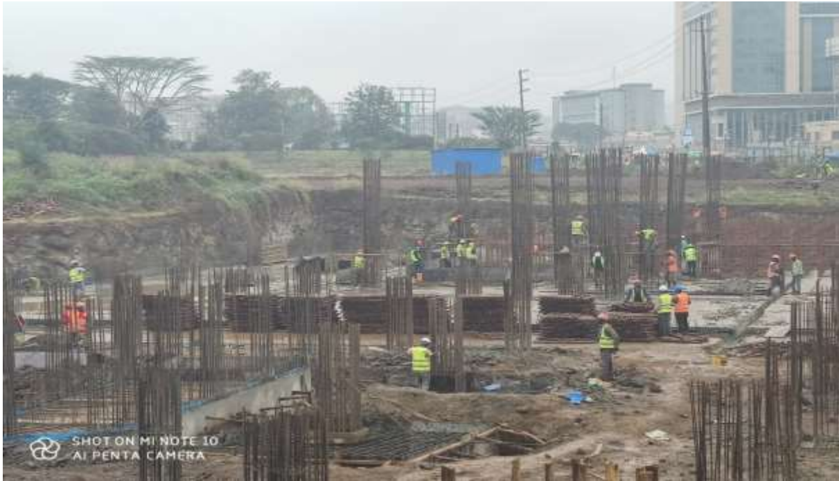
Progress in EAKI construction as at 30 th June 2020
